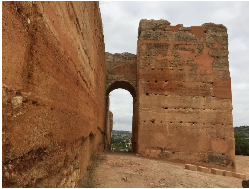
Figure 6-2 Paderne Castle in Algarve, Portugal, built in the 12th century by using earth stabilised with air lime.
