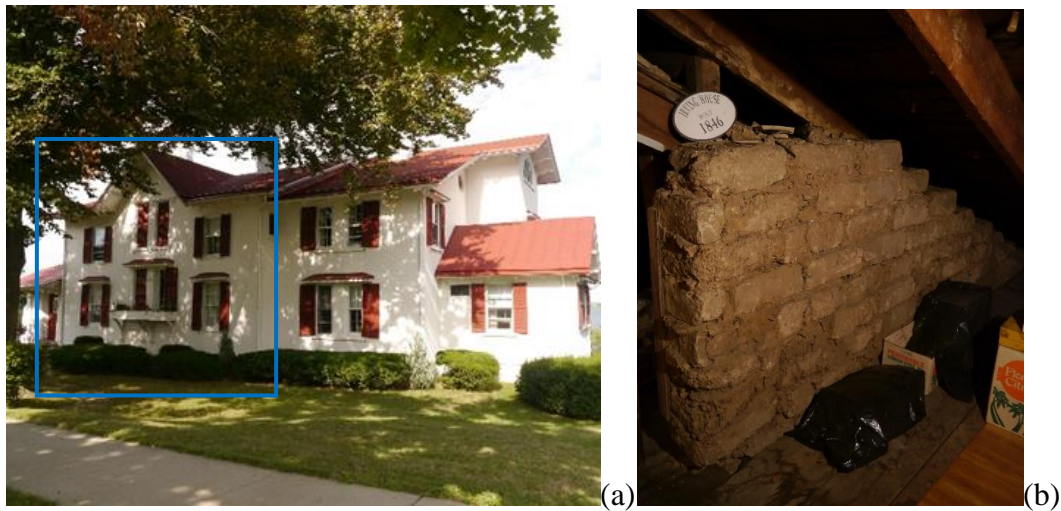
Figure 6-3 a) Irving House built in 1846 in Geneva, New York State, USA (the blue frame indicates the part built in adobe), b) adobe bricks in the attic of Irving House (Ricaud, 2014).
