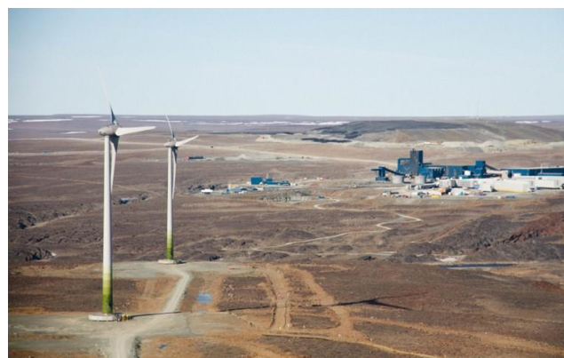
Figure 2. Wind turbines at Raglan were installed in 2014 and 2018 [29].
