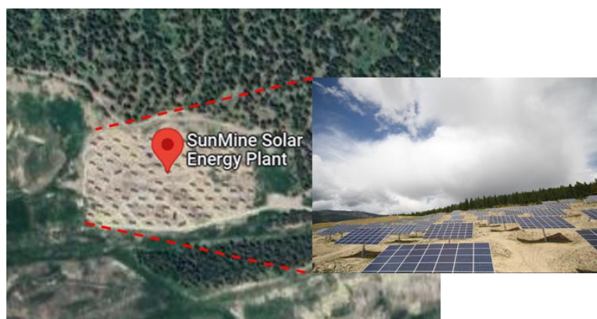
Figure 3. Aerial view of the SunMine solar energy plant in BC, Canada [31].
