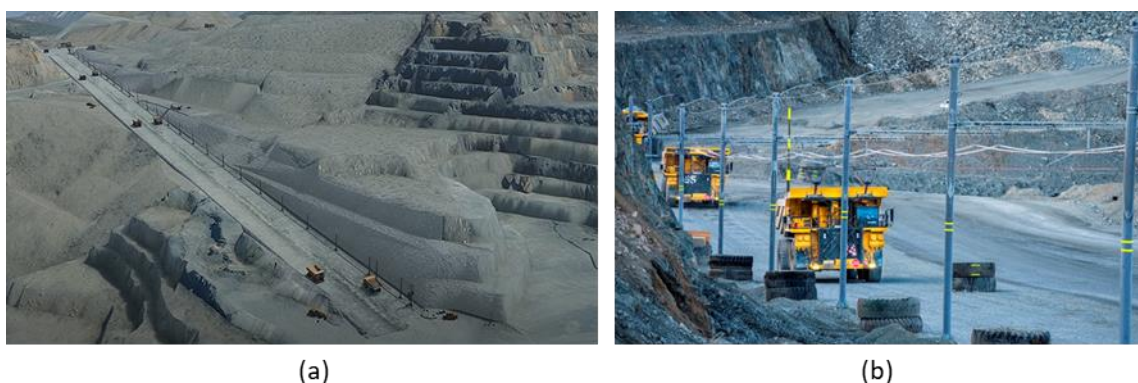
Figure 6. (a) The overall view of trolley-assist system installation at the Copper Mountain mine in B.C., Canada. (b) Haul trucks connected to the trolley-assist system network in action at the Copper Mountain mine [68].
