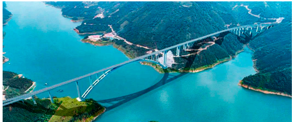
Figure 1. Tian'e Longtan Bridge constructed using CES columns, reprinted with permission from [5], 2024, www.highestbridges.com , accessed on 15 June 2024.
