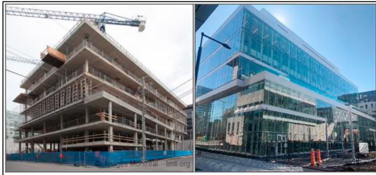
Fig. 2.1 Case Study Building Photo (MDE). Source: Ramadan, 2022.
