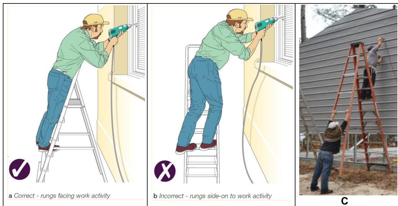
Figure 2. Stepladder with a) rungs parallel to the work, b) rungs perpendicular to the wall and c) a so named correct installation but not workable. Ref. (a) and (b) HSE; (c) US Navy Safety Center
