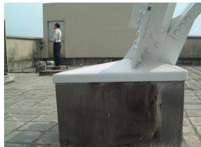
Figure 6. Tower base support for the TC1 tower
